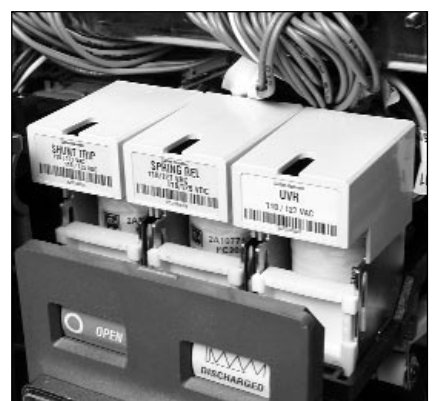
Figure 7 Shunt Trip, Spring Release and Undervoltage Release Installed
