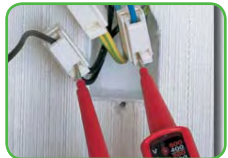
Testing through separate test slot
