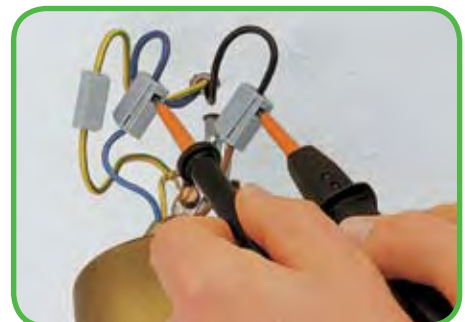
Testing through separate test slot
